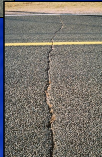
Transverse Cracking
