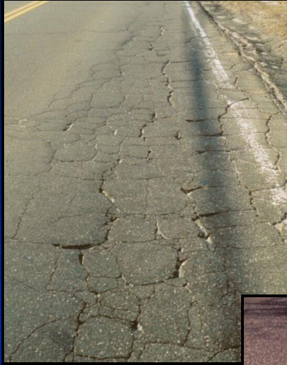
Alligator Cracking
