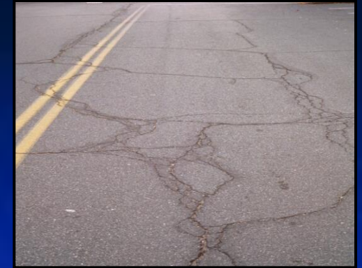
Block Cracking
