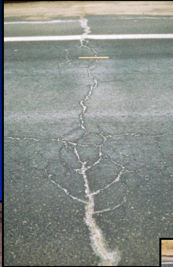
Reflective Cracking
